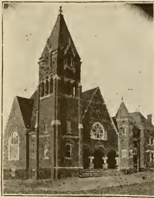
ZION EVANGELICAL LUTHERAN CHURCH, MEYERSDALE
